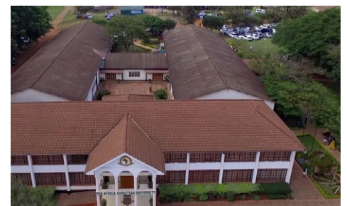
An aerial view of the main admin block of Thika Road Campus
